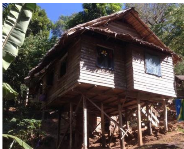
Informal settlement housing in 'at risk' area of Honiara.
